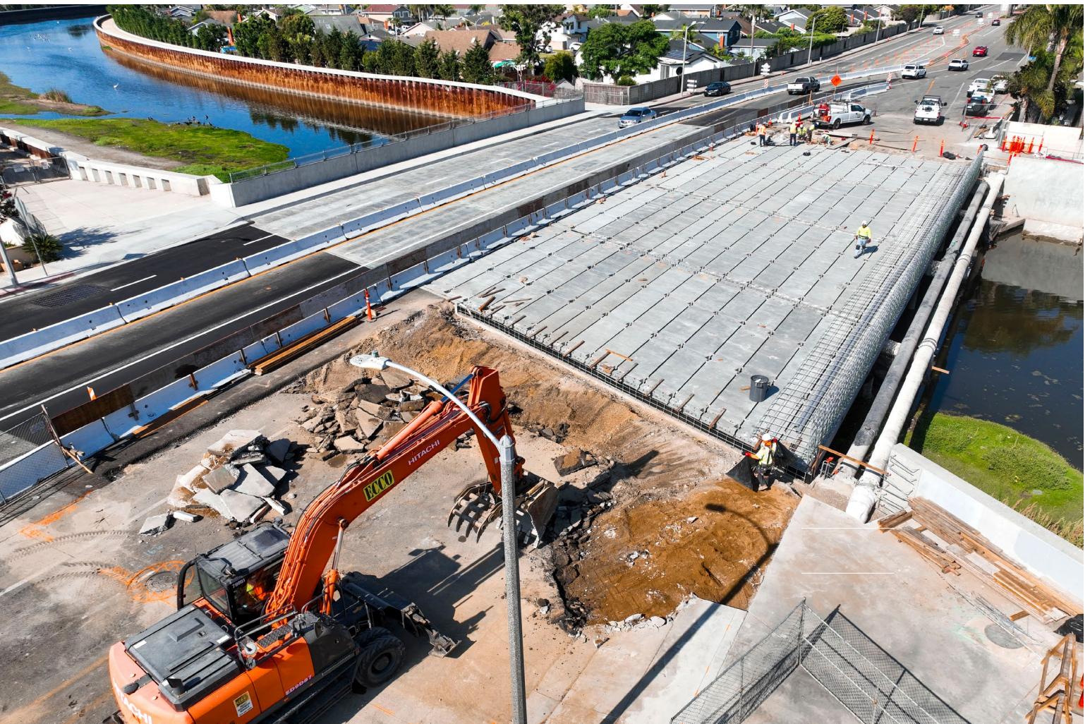
Bridge construction over the East Garden Grove-Wintersburg Channel
