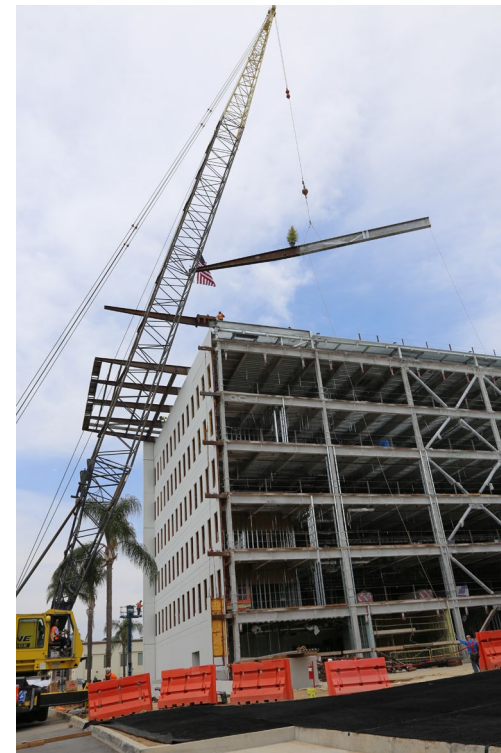
Final beam placed during construction
