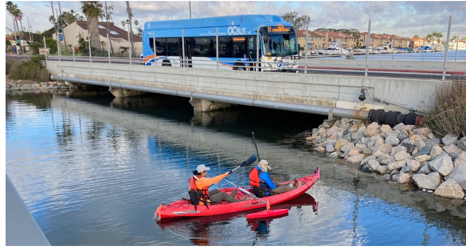
Surveyors measuring the bottom of the bay floor at the Bolsa Outlet in Huntington Beach for OC Construction
