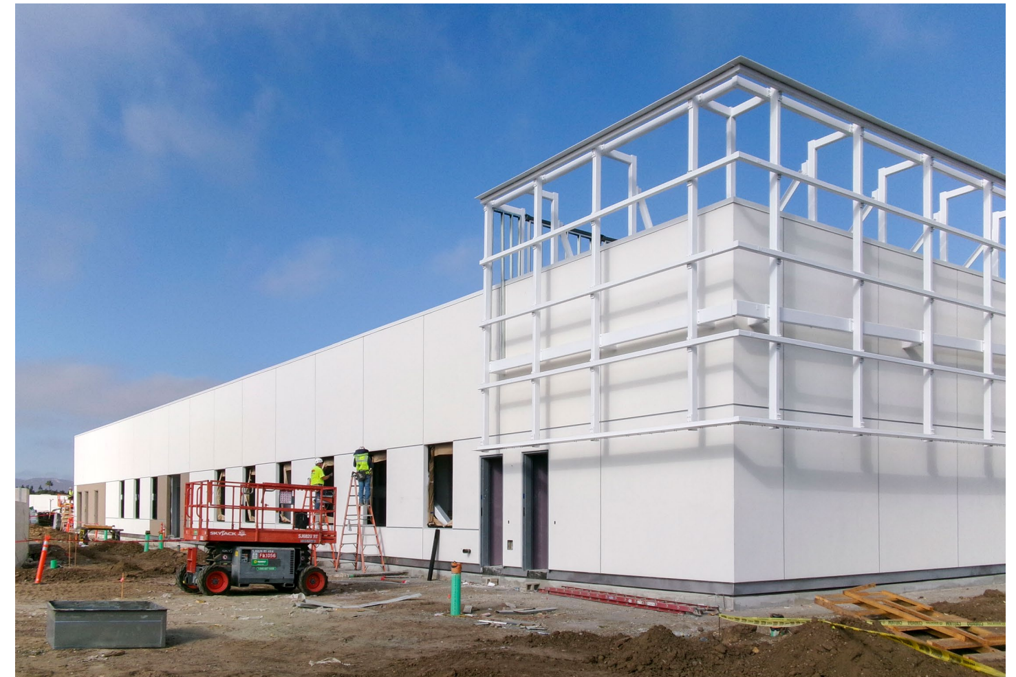
OC Health Care Agency El Toro Campus under construction
