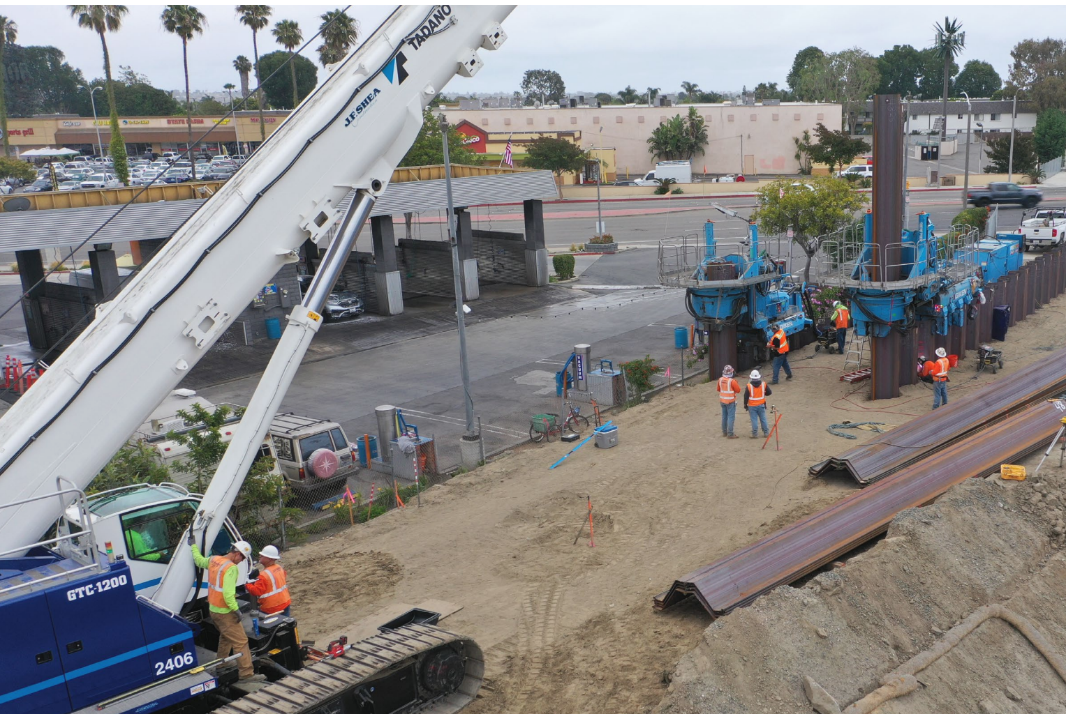
East Garden Grove-Wintersburg Flood Control Channel
