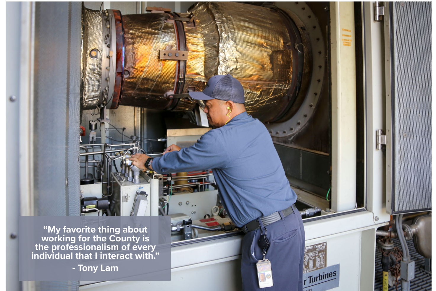
Tony monitors and adjusts the levels for the jet engine turbine that generates power and creates steam for the Santa Ana Civic Center.
