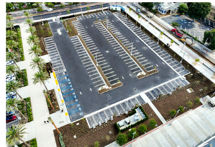
Aerial view of completed P10 Parking Lot
