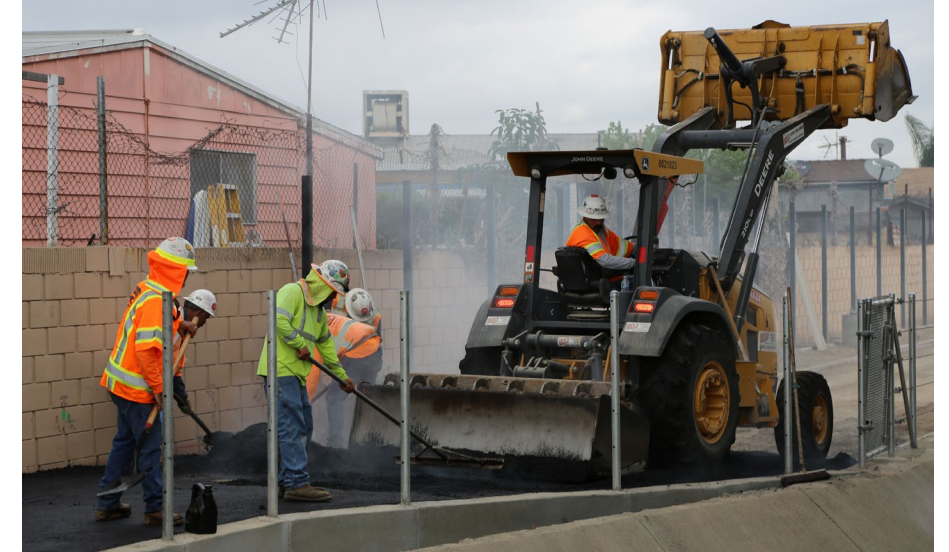
Paving the Santa Ana Gardens Bikeway Path
