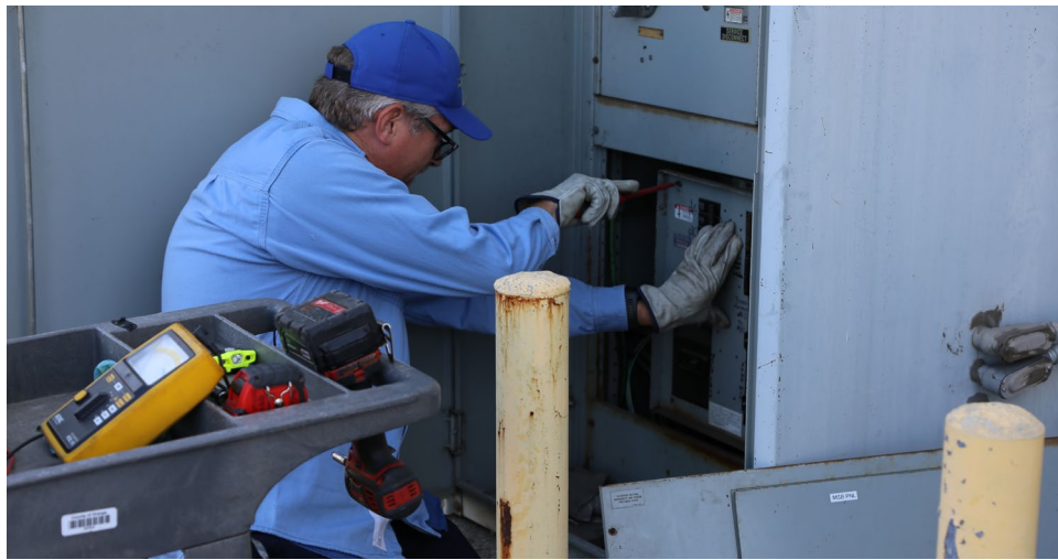
An Electrician checking the amperage of an electrical box at Fruit Street in Santa Ana
