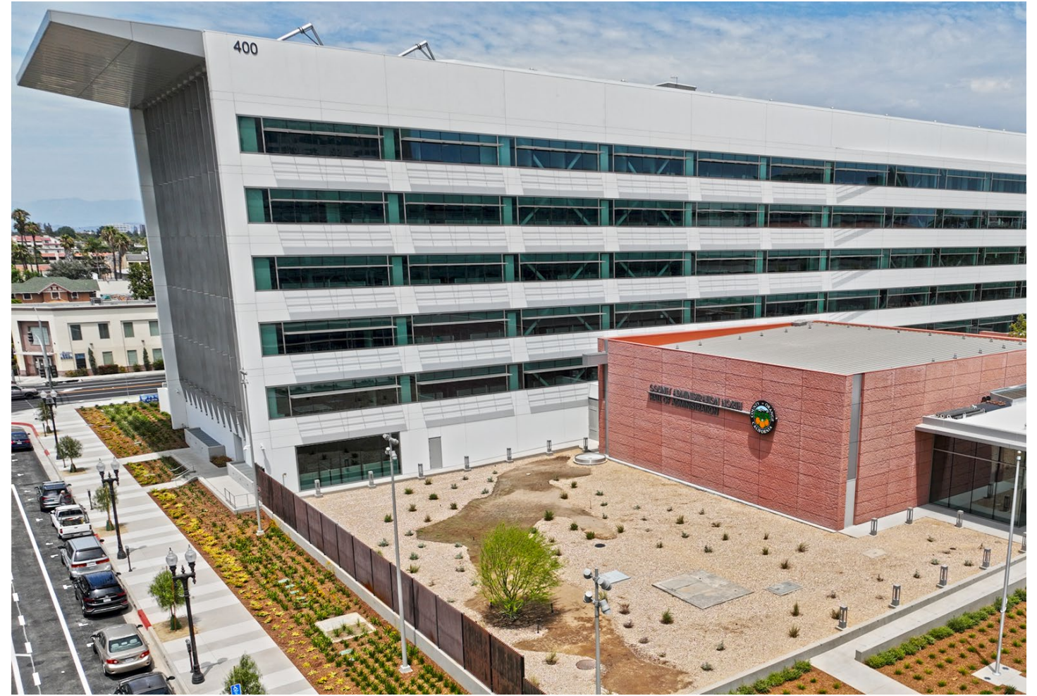
400 West Civic Center Drive, Santa Ana
