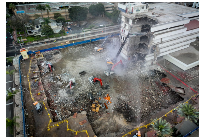
Demolition of Hall of Administration building
