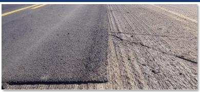
OC Public Works (OCPW) will complete a "grind and overlay" road resurfacing project to provide a smoother drive and extend the service life of streets in the North Tustin area. Access to residences may be limited during working hours, depending on the location of the work.
