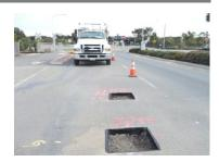
The purpose is to identify the locations of existing underground utilities, such as water, gas, sewer, electricity, phone/computer or other utility services in preparation for a future roadway and drainage improvement project.
