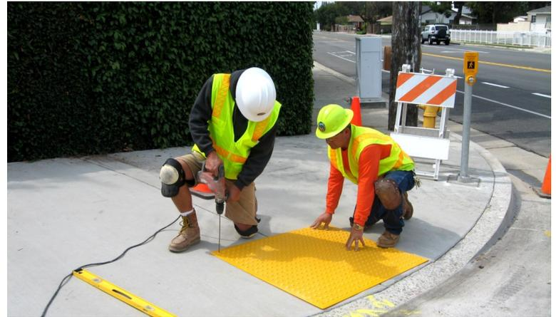
OC Public Works will be reconstructing the existing curb ramps at the corners of McFadden Avenue and Pacific Street in the unincorporated Orange County area of Midway City. The construction will upgrade the curb ramps to meet current Americans with Disabilities Act (ADA) standards. Sections of the cross gutter and spandrels adjacent to the curb ramps will also be repaired to improve drainage.
