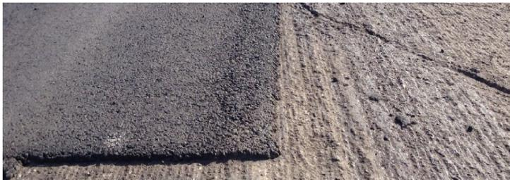
Work includes asphalt concrete overlay, utility adjustments, survey monument installations, reestablishing traffic striping and placing retroreflective pavement markers.
